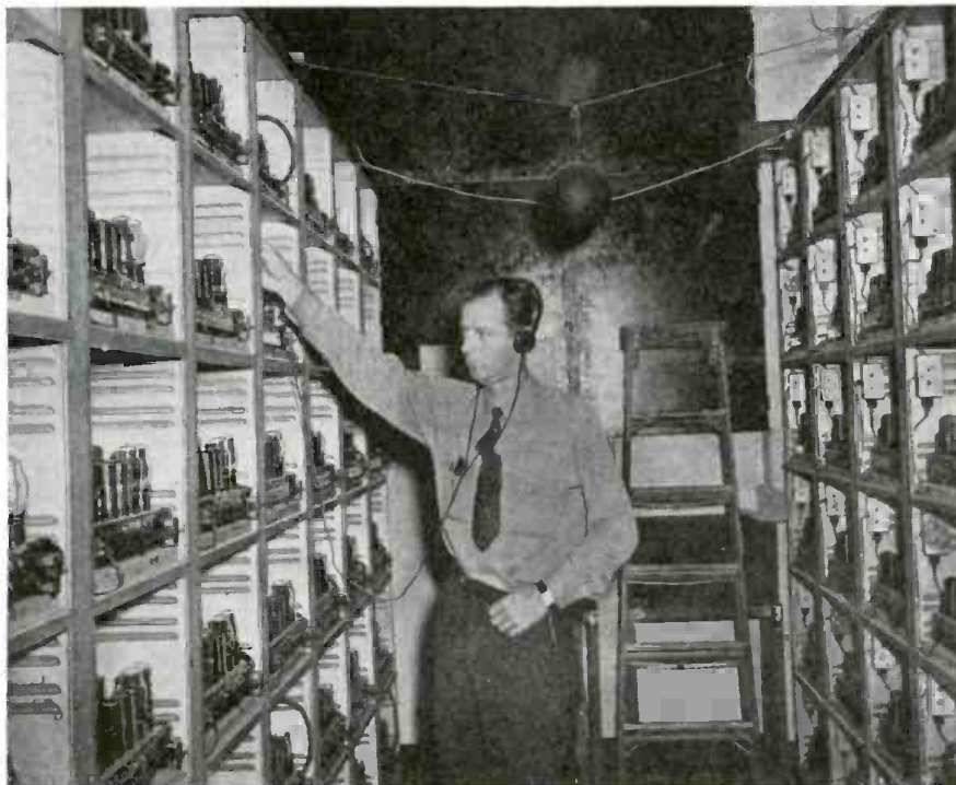
Some of the 50-watt amplifiers which furnish 5,400 watts to feed more than 600 loudspeakers. Television is Booming—Cash in on it!
