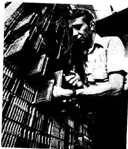
BELL LABORATORIES TECHNICIAN M. Havery inserts circuit packs in the "brain" of the No. 4 ESS System, the 1A central processor. The ribbon-like strips snaking down the front of the control unit are actually cables connected to test equipment.
