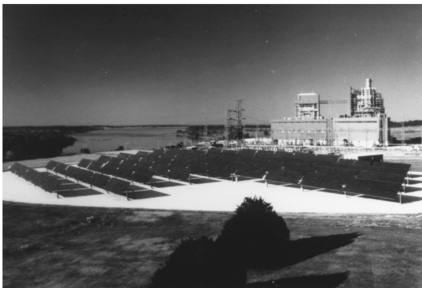
FIGURE 60.2 A view of the city of Austin PV-300 flat-plate grid-connected photovoltaic system. (Courtesy of the city of Austin electric utility department.)
