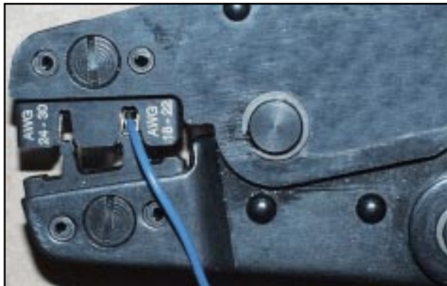
(3) The stripped wire is placed into the terminal and crimped. Note the wire's insulation must stop just short of the conductor tabs (detail)
