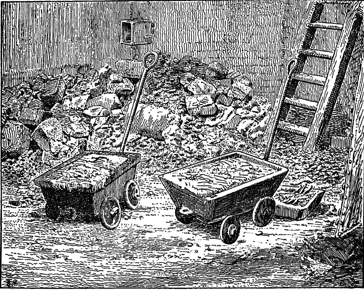
Fig. 68.—Tapping cinder from ball furnace.
