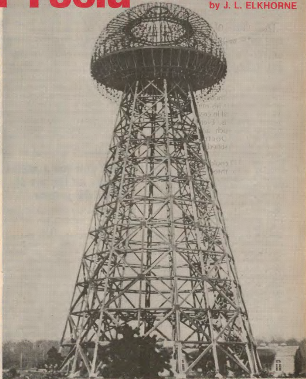
This tower was built on Long Island in 1904 while Tesla was experimenting with power distribution by wireless.
