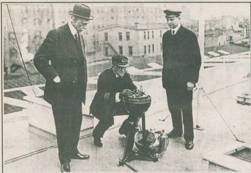
Sperry examining the repeater compass for his gyrocompass installation aboard the Princess Anne, 1911.
