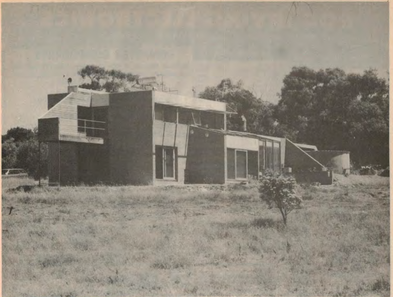
The house is oriented east-west with the front facing the northern sun to maximise energy gain and minimise heat losses.
