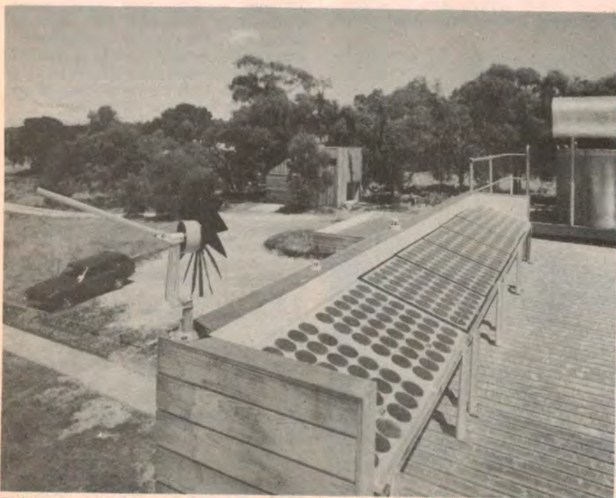
Eight solar cell arrays each provide 2.5A at 14.5V, with a total capacity of 20A.
