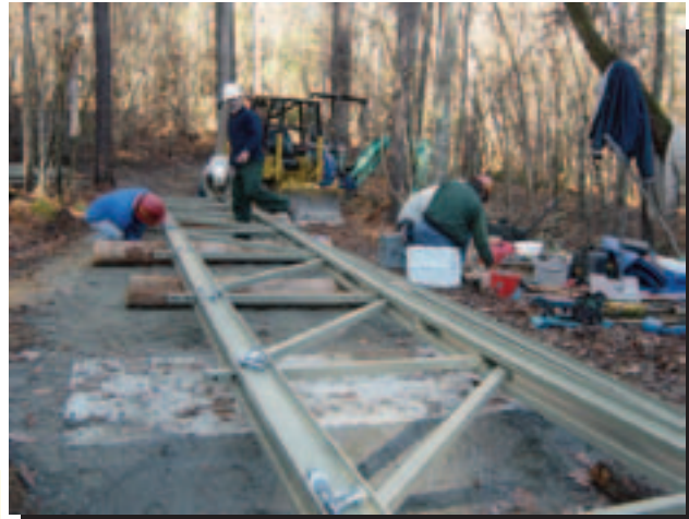
Figure 17—Assembling a truss on level ground near the bridge site.
