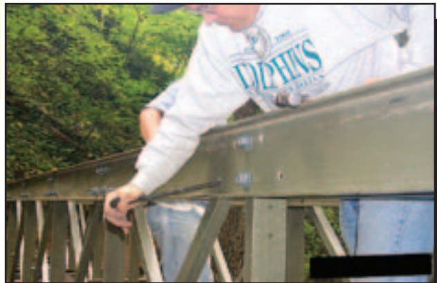
Figure 18— A tapered bar can be used to align bolt holes.
