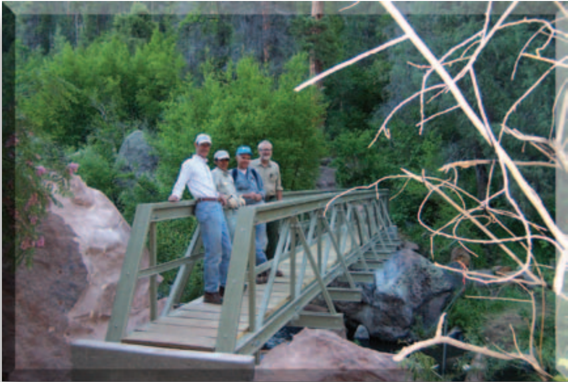
Figure 1—A fiber-reinforced polymer trail bridge in the Santa Fe National Forest.
