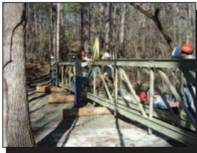
Figure 19—Trusses are set upright before being moved into place.
