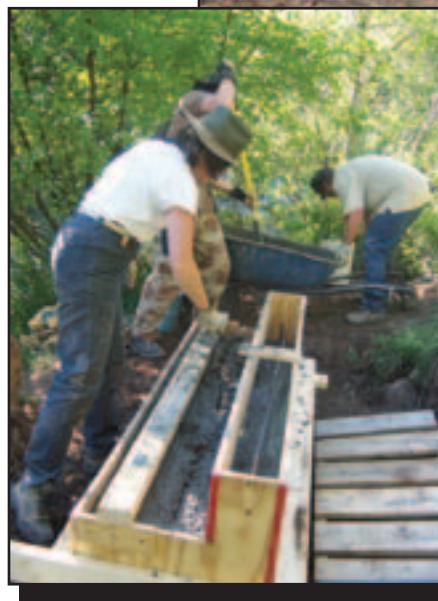
Figure 16— Constructing an abutment for an FRP bridge.
