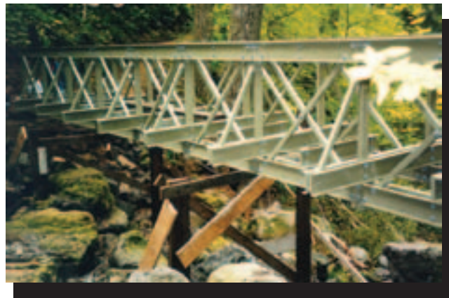
Figure 13—Sometimes, temporary supports must be used when constructing longer bridges.
