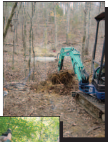
Figure 15— Clearing an abutment with a small trackhoe.
