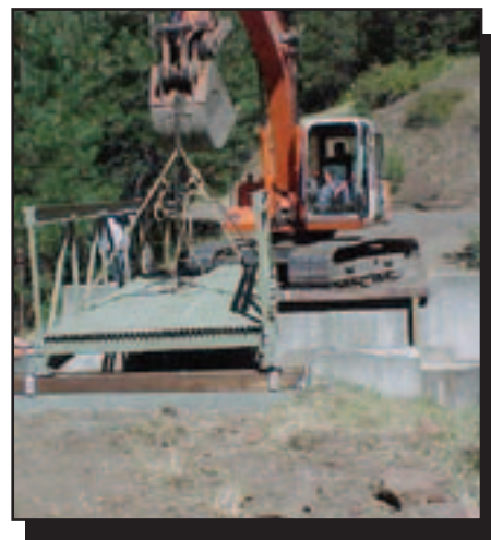
Figure 10—A track hoe placing a trail FRP bridge on its abutments.
