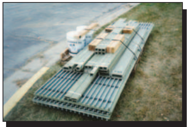
Figure 34—The materials for an FRP bridge after delivery to the Forest Products Laboratory.
