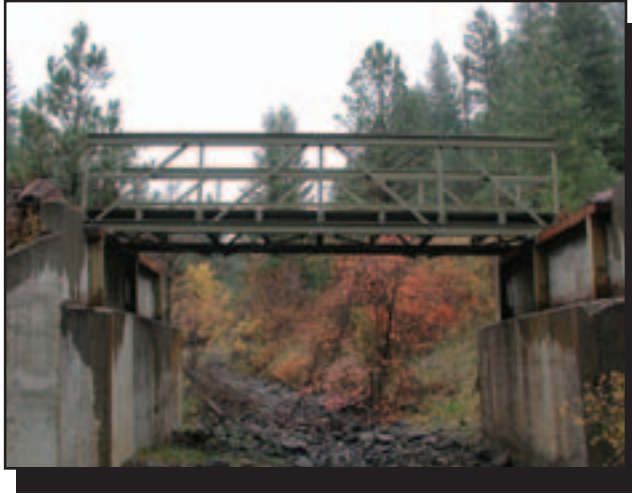
Figure 46—A side-truss FRP bridge in the Wallowa-Whitman National Forest.
