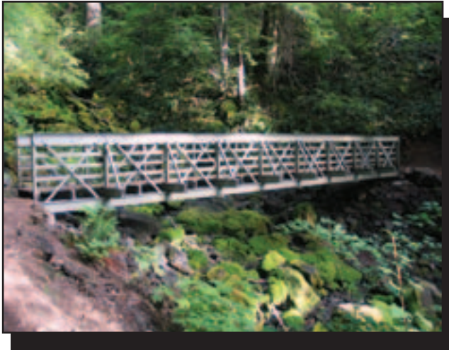
Figure 42—A side-truss FRP bridge in the Gifford Pinchot National Forest.
