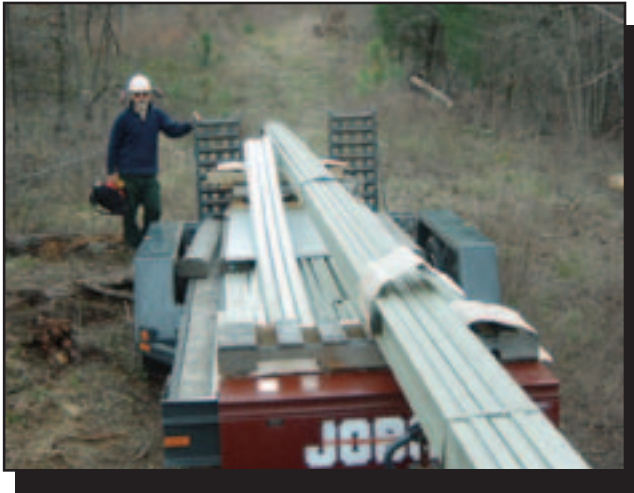
Figure 11—FRP bridge materials being delivered to a staging area.
