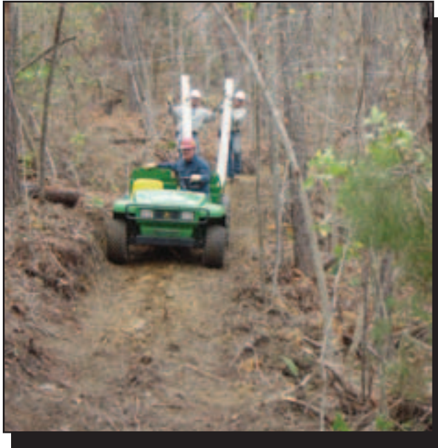
Figure 5—FRP members are lightweight and can be lifted by hand.
