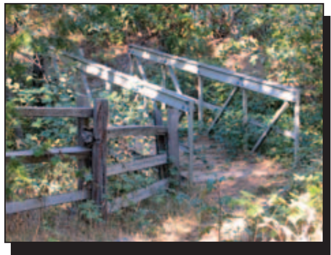
Figure 48—A side-truss FRP bridge in the Tahoe National Forest.
