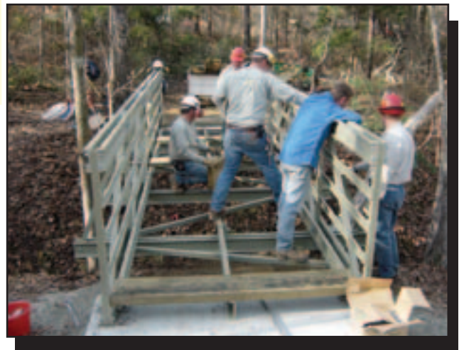
Figure 21—Installing and fastening cross bracing.
