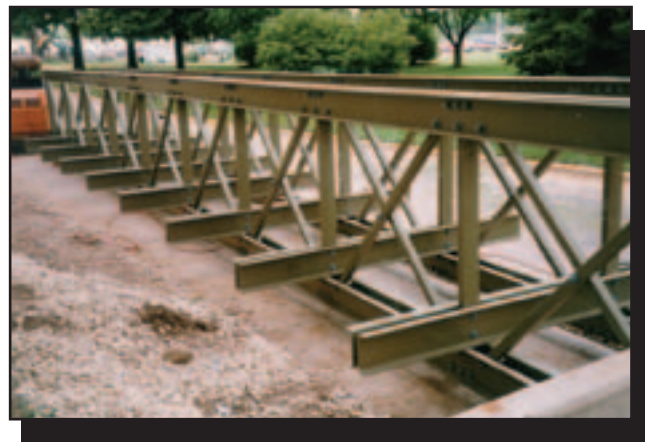
Figure 37—Disassembling an FRP bridge after testing at the Forest Products Laboratory.
