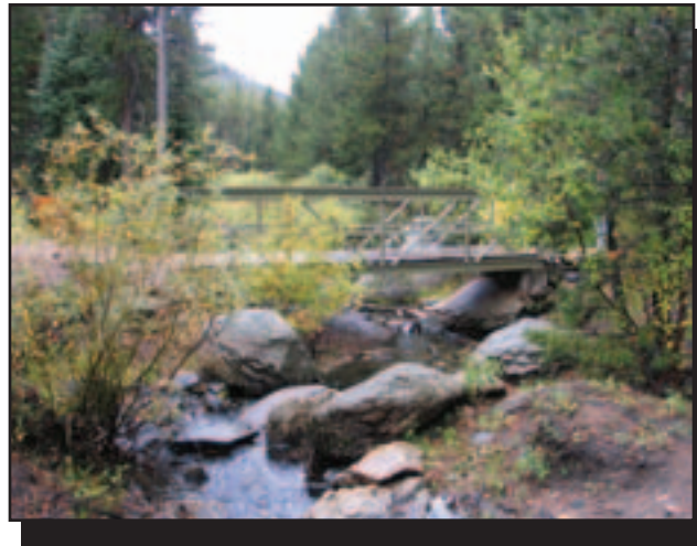
Figure 44—A side-truss FRP bridge in the Medicine Bow-Routt National Forests.
