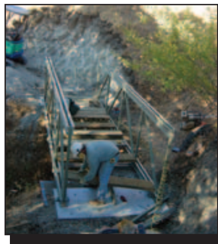
Figure 22—Fastening deck planks.
