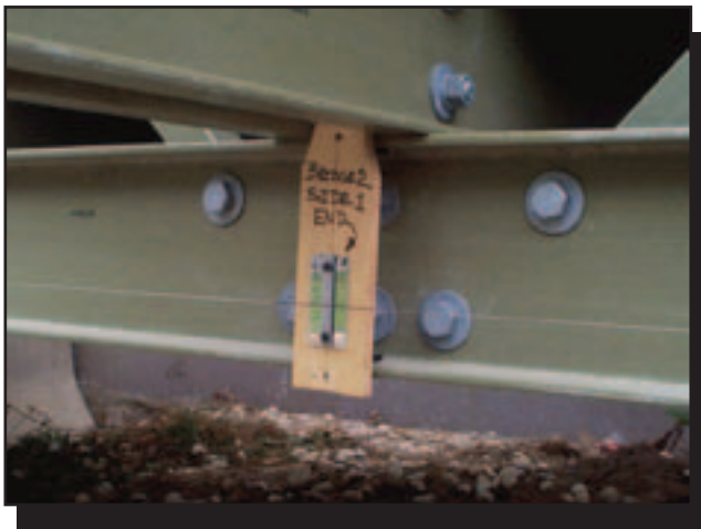
Figure 35—The typical setup of a deflection gauge used to test bridges.
