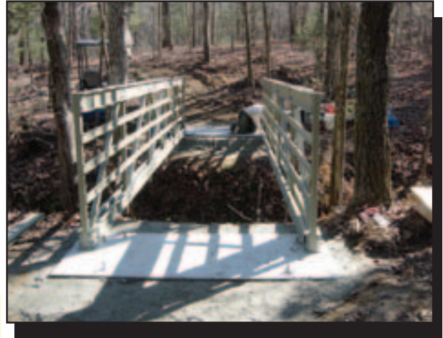
Figure 20—Squaring up bridge trusses.
