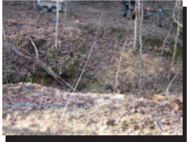
Figure 14—Staking out a bridge site with a cloth tape.
