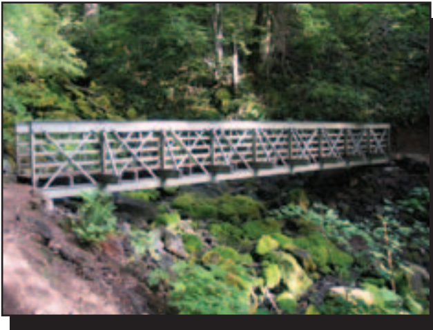
Figure 8—A side-truss FRP bridge in the Gifford Pinchot National Forest.
