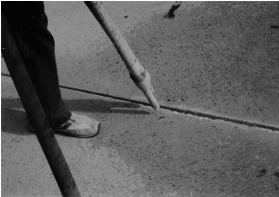
Figure 10.3. Sandblasting a joint face
