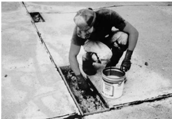
Figure 16.1. Application of bonding agent to the concrete surface. Note the joint filler bordering the repair area
