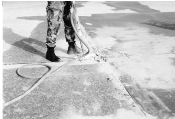
Figure 14.2. Using a jackhammer to remove damaged concrete
