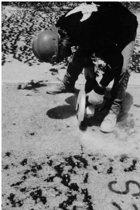
Figure 10.1. Hand sawing a crack
