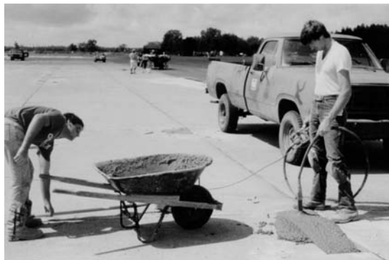
Figure 16.2. Consolidation of the repair material by vibration
