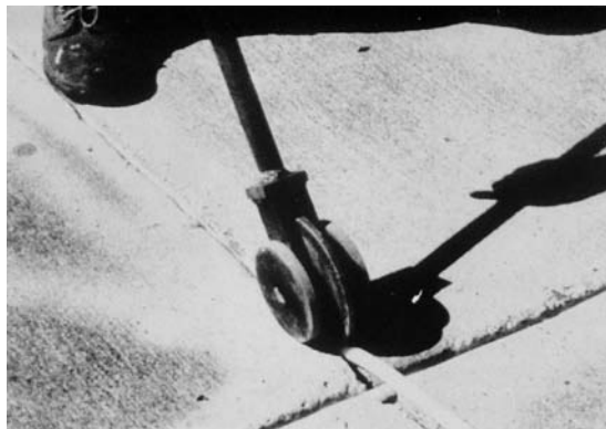
Figure 9.6. Installation of backer rod
