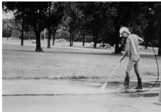
Figure 9.4. High-pressure water cleaning
