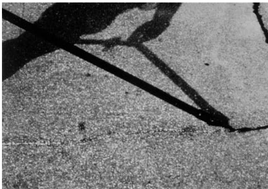
Figure 11.1. Sealing a crack
