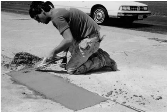
Figure 16.3. Finishing the patch surface
