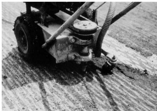
Figure 9.2. Vertical spindle router
