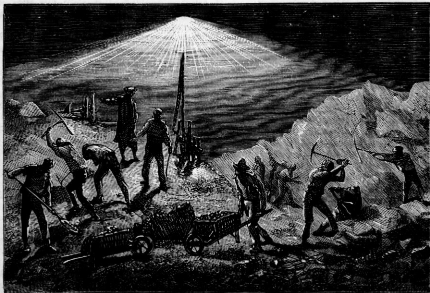
NIGHT-WORK BY ELECTRIC ILLUMINATION.
