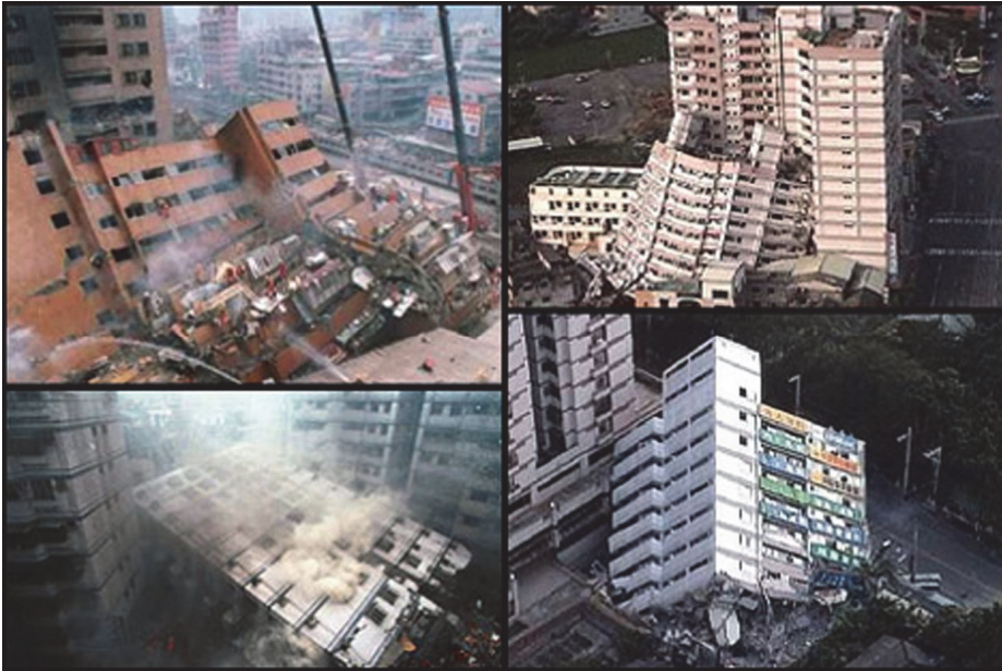
Fig. 1. Damage to buildings subjected to strong earthquakes, (9-11 Research Book, 2006)
