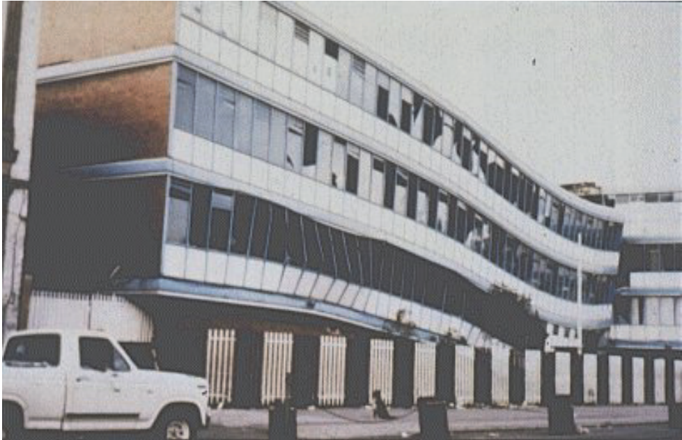
Fig. 2. Mexico City building failure associated with the torsional-translation motion, (Earthquake Engineering ANNEXES, 2007)
