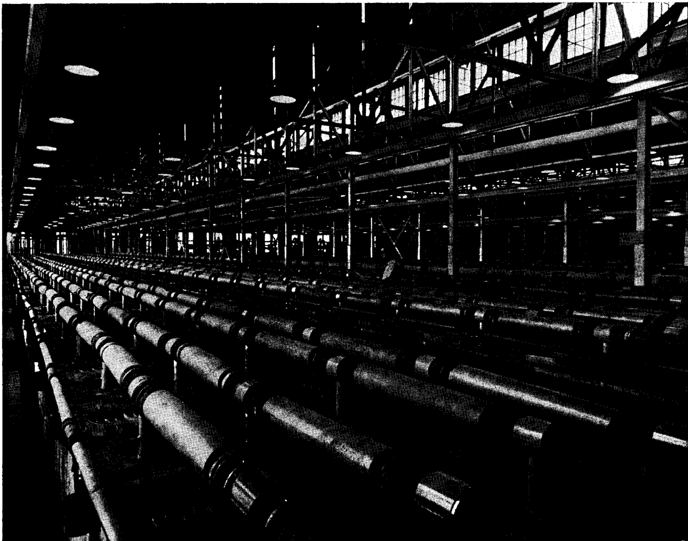
LARGE ELECTROLYZER PLANT for the production of hydrogen by the electrical decomposition of water is operated by Cominco, Ltd., in British Columbia. The 3,200 electrolytic cells, which
