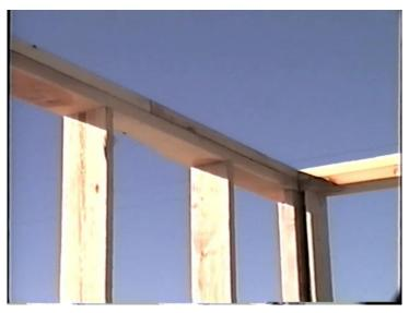
A top plate all the way around the exterior wall will be a 2x4 or a 2x6 depending on the thickness of the wall. Most interiors are 2x4 studs so the top plate will be 2x4's. Make sure to offset the joints to maintain stability. See **figure 4.18**
