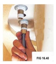
You will need two supply tubes. These tubes come in different lengths and they come in plastic or metal. They have fasteners at each end so they can screw onto the sink intakes and the plumbing waterlines as shown in **figures 16.39** and **16.40**.
