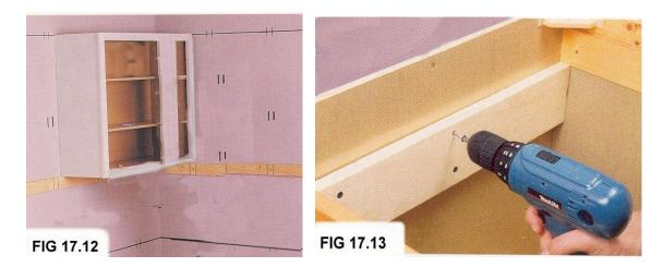
As shown in **figure 17.12**, the first wall cabinet is resting on the board or sometimes called a ledger to help hold it until all the screws are put in. It's very important to get a good hold. The size of screws to use depends on the wall stud or joist it's going into. Most cabinet installers use 3 or 4-inch screws. See **figure 17.13**.
