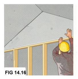
A T-square can help make perfect cuts for straight pieces as shown in **figure 14.15**, but a chalk line is usually the best tool for tricky cuts as in **figure 14.16**.
