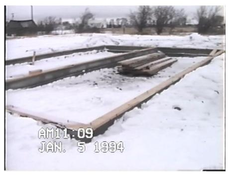
After the foundation was finished we put the sill plate on all the way around and bolted it down. We kept the old forms, which we used for the foundation cement work. We'll use them for the floor joists to save money. It's kind of hard to see with all the snow. It slows down the work progress at times, but at least you don't get too sweaty!
