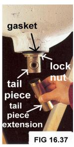
As we can see in **figures 16.36** and **16.37** the drain connects with the tailpiece. The tailpiece is held onto the sink with the underside locknut. The tailpiece extension then goes into the p-trap.
