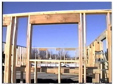
After you get the walls up, you will need to run a double plate on top to hold the sections together better. The same thing applies to the interior walls. See **figure 4.17**
