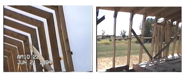
On the left, you can see the knee without reinforcements. On the right, the knees have been reinforced on each side with 2X6's. The angle on these knees are not within code because of the weak pitch; however this roof will have a dividing support wall to brace the rafters up bringing it into code.
