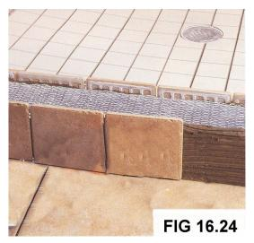
Lay out another layer of mortar while keeping in mind that the tile needs to be just slightly above the drain when it's installed. This will help us remember how high to make the mortar. Let this dry overnight and then we can start with the tiles. It's easier to get the sheets of tiles than to do one at a time. From this point, it's just a matter of securing the tile and grouting in the cracks. See **figures 16.25** and **16.26**.
