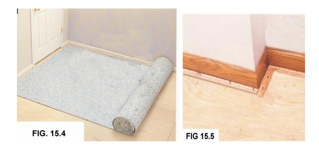
You will need the carpet pad, which goes down first. See **figure 15.4**. You will need to nail all the tack strips in place, which actually holds the carpet in place without having to use tacks. The tack strip will be placed <sup>1</sup>/<sub>4</sub>-inch away from the walls. See **figure 15.5**
