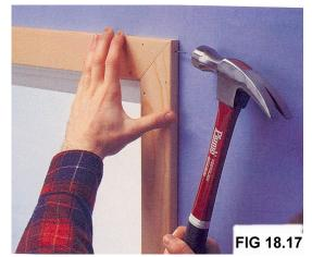
The window trim is almost as easy as the door trim except you have four sides and they all need to match up so you don't have big cracks between the trim pieces. Silicone can only do so much. **Figures 18.16** and **18.17** show how to attach the window trim for perfect 45-degree angles. **Figure 18.18** shows a slightly more complex angle, but still very easy to figure out. The octagon window has been such a big hit with my children.
