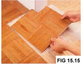
Tap them gently with a piece of scrap wood and a hammer to make them fit tightly together as shown in **figure 15.14**. You can make special cuts for the final tiles with a jigsaw or a coping saw and place them in until you have a perfect fit. See **figure 15.15**.
