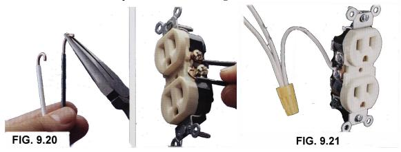
Tighten down the screws really well. Most receptacles and switches have insertion fittings or holes on the back to put wires in. This gives more options, but seldom do electricians use the insertion fittings because it crowds the wires inside the box often causing wire connectors to come apart. Most electricians use the screws on the side of the receptacle.
