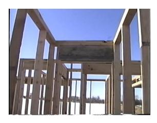
When you put each piece of wall up, there is a danger that it could still fall down or even get blown over by the wind. They are heavy and need to be braced until the outside sheathing is applied. **Figures 4.22** and **4.23** show how this is done.
