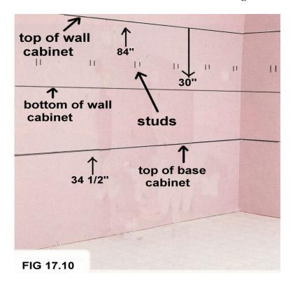
It makes the job easier if you mark a level line where the top of the wall cabinet will be. From there you can mark where the bottom of the wall cabinet will be. If you're short on help, you can put a 1X4 where the bottom of the wall cabinet will be and it will help support the weight of the cabinet until you get it completely fastened down. See **figure** 17.11.
