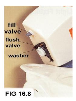
**Figure 16.8** shows how the tank will fit on to the toilet and where the screws need to be secured. **Figure 16.9** shows where the bolts will be tightened and **figure 16.10** and **16.11** shows the connection of the waterline and the toilet seat. And that is it.
