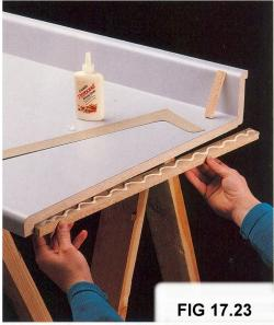
The post form countertops are already made so you just cut them to the right length and put a batten in the end. The batten helps make a more secure end plate. See **figures 17.22** and **17.23**.
