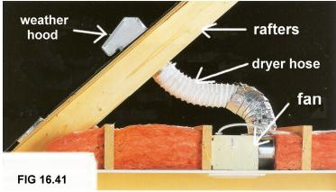
You'll first need to cut a hole in the roof the size of the vent flange. The vent cover will completely cover the hole and the flange will stick into the hole and connect to the dryer vent. See **figure 16.42**. Connect the dryer vent with a hose clamp as in **figure 16.43**.
