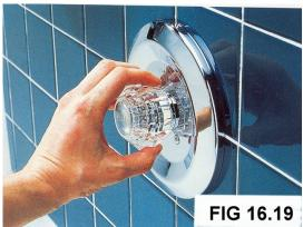
Every building center has the right parts for shower and bath anti-scald valves so don't worry about getting the wrong parts. It would be difficult to find shower pipes without anti-scald valves these days. The shower handle assembly comes with a cover that fits into the cut out hole in the surround. The top of the handle comes off and under it is a screw for tightening the handle. You just pop the top back on when it's done.
