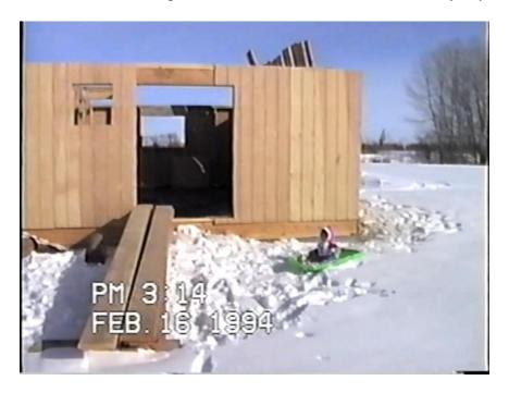
When you get to the windows and doors, you can either piece together strips of sheathing or just cover up everything and use a router to cut them out. I like to keep the sheets big because it gives more strength. You can use a jigsaw or a saber saw to cut things out either. If you are using plywood, you might consider running the sheets sideways so that the wood grains give more strength.
