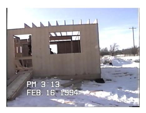
I used a sheathing called T-111. Initially I wanted to save money by using a sheathing that could be painted to save on vinyl siding costs. That was a dumb idea because I really hate to paint. It was sort of an expensive lesson, but it worked out fine anyway.
