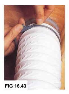
Connect the other end of the dryer vent to the fan outlet using another hose clamp. The wiring should have been run with the electrical so it's just a matter of connecting the hot and neutral wires. See **figure 16.44**. Some fans are a fan, heater, and a light. In this case you will have three sets of wires to keep straight and run to a switch or switches as we've covered in chapter 9. Remember that all bathroom outlet switches need to be GFCI's. See **figure 16.45**
