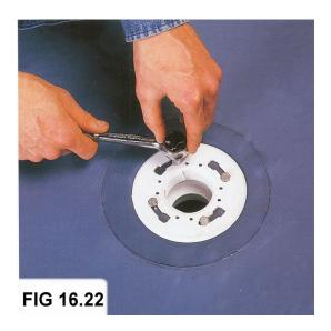
You can reinforce the membrane over the drain if you want to for more strength. Now screw the middle drain piece down evenly and tightly to make a watertight seal. See **figure 16.22** Next, we put the backer board on the walls and put the third drain piece in.
