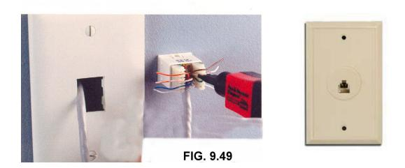
You'll need a special tool for terminating RJ45 network cables. See figure 9.50
