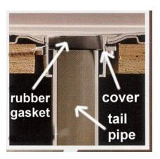
Now let's lay the mortar to show how it needs to be done. The shower pan should be ready to put in place. Make sure you have the drain cover, rubber gasket, and tailpipe installed and it is tightened down with a drain collar nut. See **figure 16.14**
