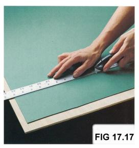
You will want to cut the sidepieces because they will go on first and try to leave extra to get routered off. See **figure 17.17**. The laminate is attached to the countertop with contact cement and pressed in place. See **figure 17.18**. Once it has had a short time to dry, you can router off the edges using a flush-cutting bit. See **figure 17.19**.
