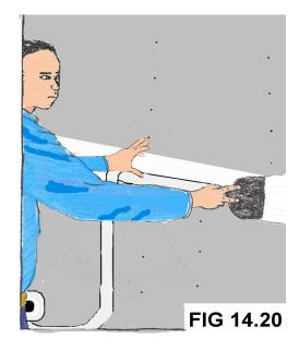
You will want to make sure that the tape is exactly the length that is needed because splicing the tape makes a seam that's hard to cover. As you squeeze the compound out from under the tape, make sure to get all the wrinkles and blisters out. If you get blisters or little round bubbles in the tape, you probably aren't getting enough compound on the wall before the tape goes on.
