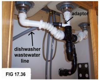
If you have a dishwasher you will need to have an outlet for the wastewater. A good place for that outlet is right on the tailpiece on the sink assembly. You can get tailpieces with dishwasher adaptors at any plumbing store. Almost everyone has a dishwasher these days. See **figure 17.36**
