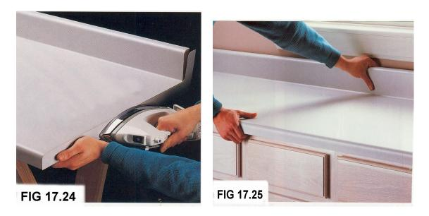
When putting the end cap on you will need to activate the adhesive with an iron so it will make a good contact. See **figure 17.24**. Post form countertops are almost a guaranteed success. They make the job very easy.
