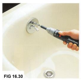
The overflow is attached by inserting two screws through the overflow plate and the drain is secured by screwing it into the drain waste assembly to make a water tight seal See figure 16.30.
