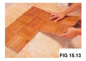
After you've marked the floor then you can apply the flooring adhesive with a notched trowel. The adhesive dries fairly quickly so you might want to cover only as much of an area that you can work on inside of an hour. See **figure 15.12**. Next you will start laying the tiles in place according to the measurements on the floor. See **figure 15.13**. Some types of floor laminates need to be glued. Once in place, make sure they fit tightly together.
