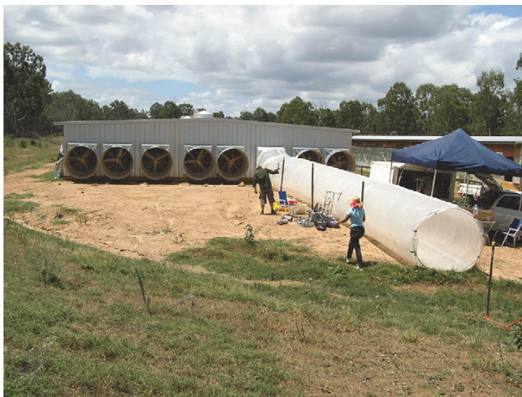
Fig. 4. Tunnel ventilated broiler shed showing polyethylene sampling duct attached to an exhaust fan. (Sohn et al., 2008)
