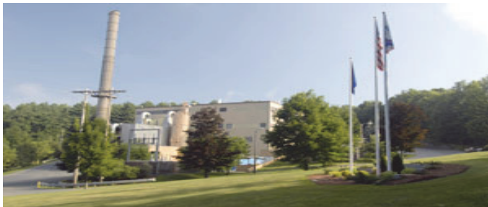
Fig. 6. Wheelabrator Technologies, Inc., Claremont, NH.
