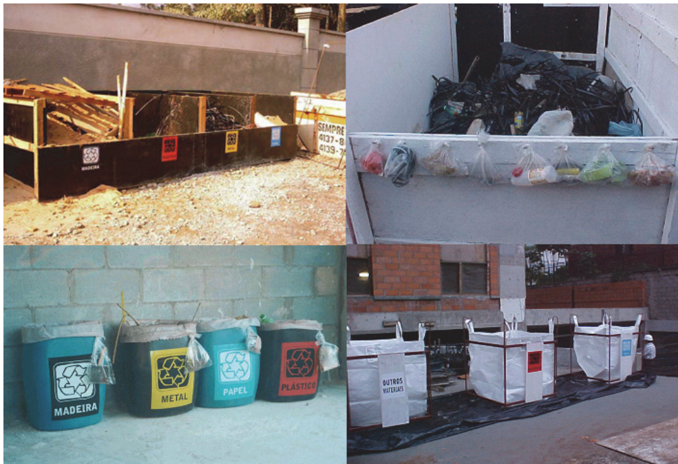
Fig. 4. Segregation of waste at the construction site
