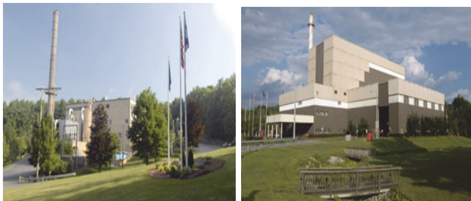
Fig. 7. A and B. Wheelabrator Technologies, Inc. in Claremont and Concord, NH, respectively.
