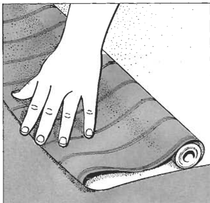
4 Fold the roll back on the paper you just measured. Crease the paper at the small cut and use it as a cutting guide.
