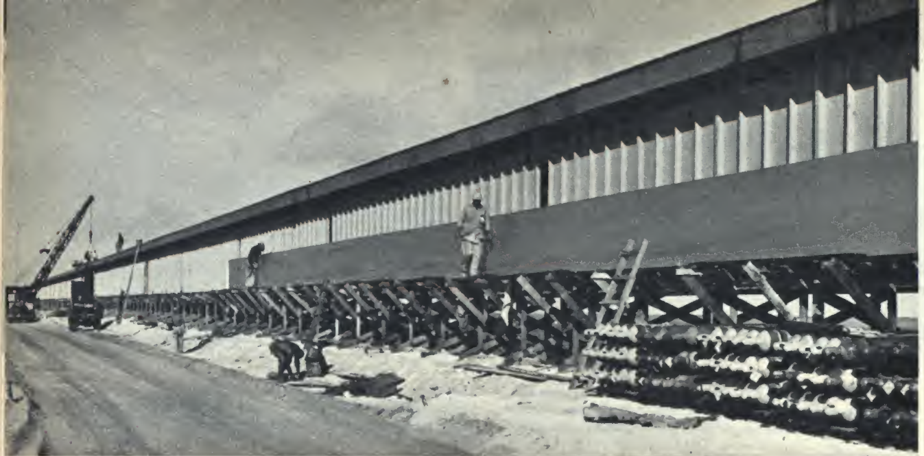
Here is a plywood tube running from Elugelab for two miles to Bogon, most of it within fireball area.
