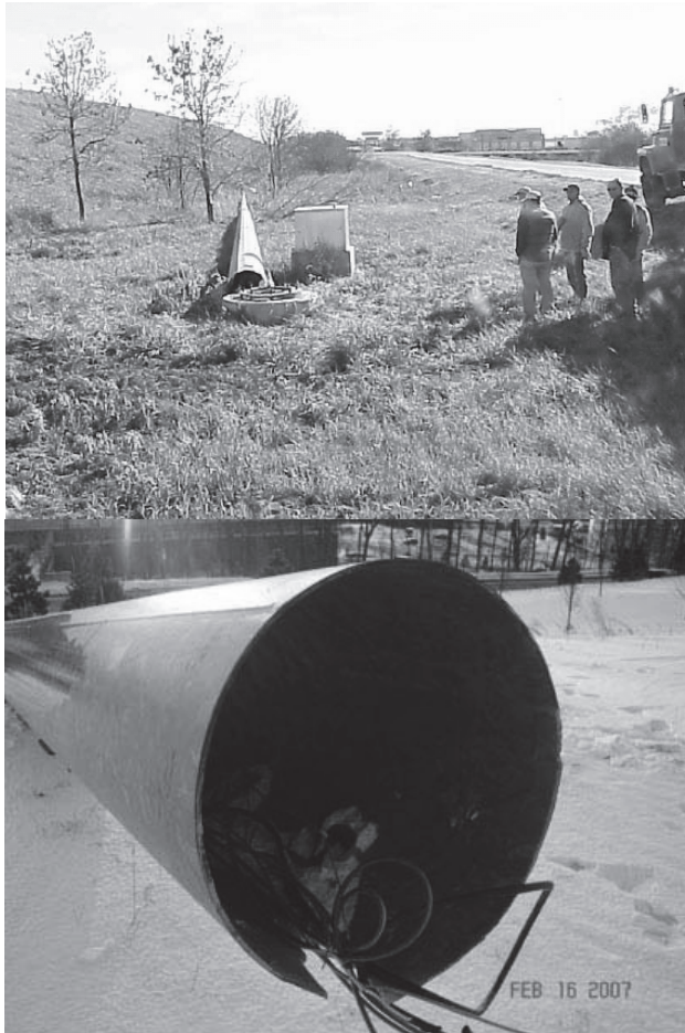
Fig. 1. A collapsed high-mast light pole; (a) Iowa (Dexter 2004), (b) Colorado (Rios 2007)
