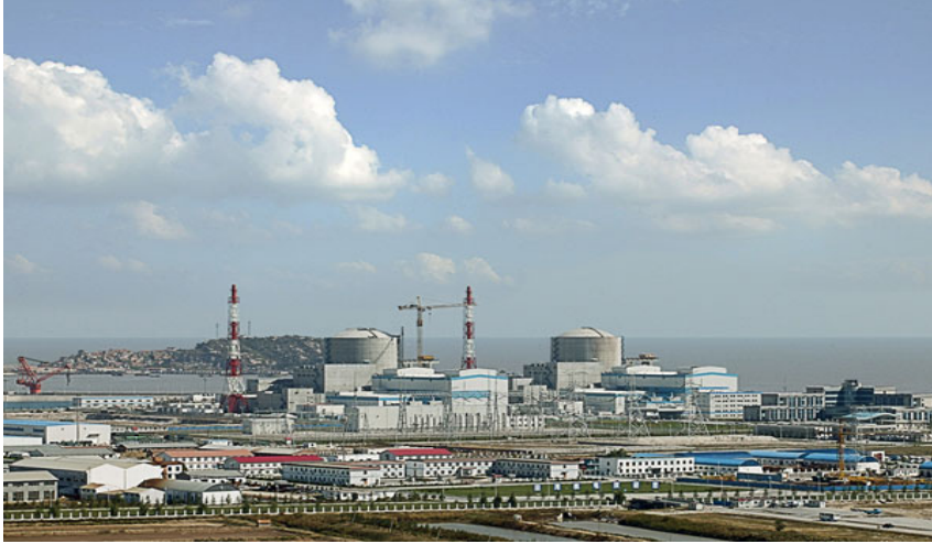
D: Tianwan Nuclear Power Plant in China (From http://www.heneng.net.cn/ )
