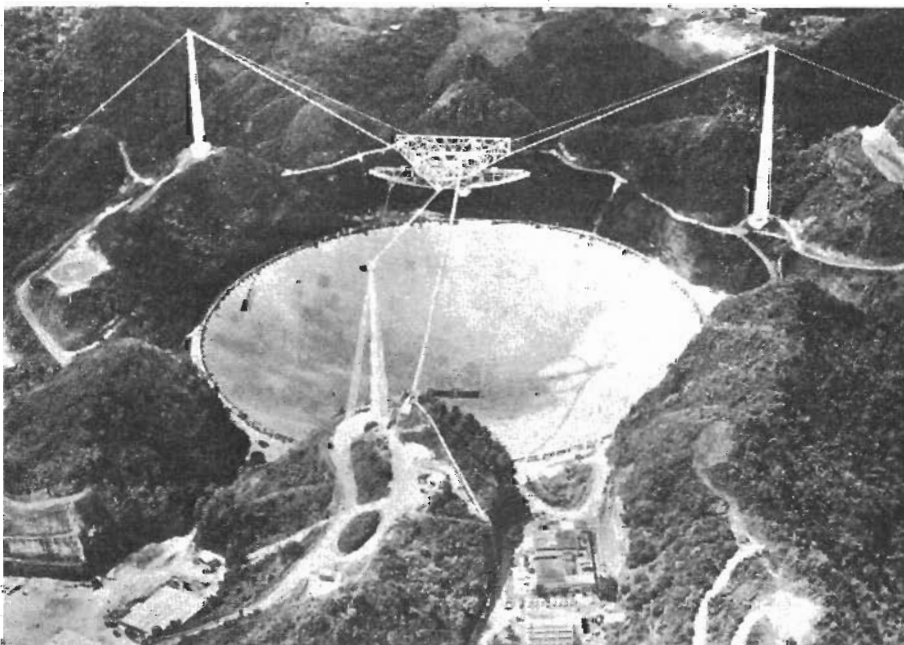
Fig. 1. The radio telescope at Arecibo, Puerto Rico. The paraboloidal reflecting dish, 300m in diameter, is constructed within a natural valley in limestone mountains. The feed is supported 137m above ground by cables attached to three pillars. By moving the feed the telescope is made semi-steerable (at 1.42GHz, to any direction within 20° from the zenith).
