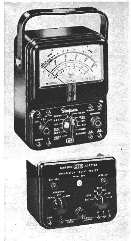
Model 260 multimeter and 650 transistor-tester adapter.
